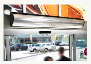
In 2013, the LDB specified that air curtains must be installed over sliding front doors in BC Liquor Store locations to create a barrier between indoor and outdoor air and improve the efficiency of heating/cooling systems. Air curtains were installed in 15 existing BC Liquor Store locations in 2014. Three new locations which also opened in 2014 had entryway vestibules installed to create an even more effective barrier between indoor and outdoor air.
