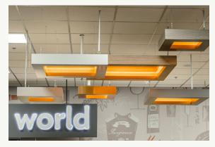
Six renovations and construction projects completed in 2014 used very efficient LED fixtures for general overhead lighting. This new lighting is now standard in the LDB's specifications handbook for building contractors.
